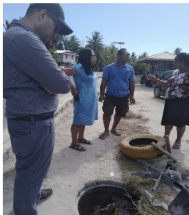
(a) Manhole access to existing duct
